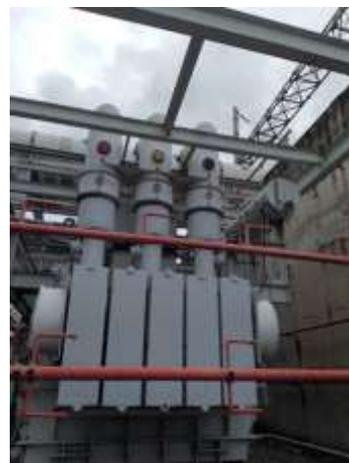
**Gambar 7 Transformator UAT A**
