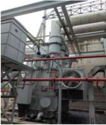
**Gambar 8 Transformator UAT B**
