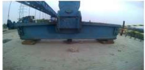
Gambar 13. Pemasangan *Hanging Beam*
