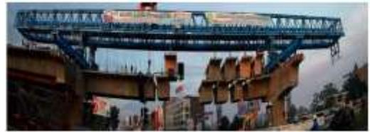
Gambar 6. *Lifting gantry*
